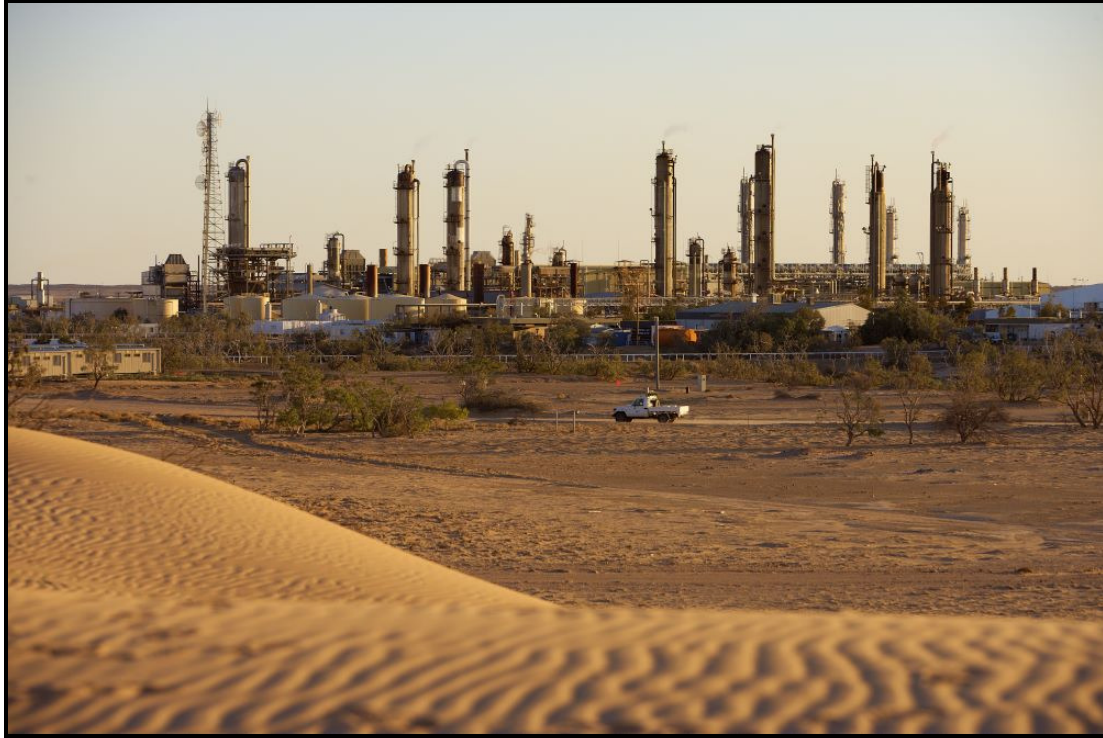
Figure 2: The Moomba Gas Plant
